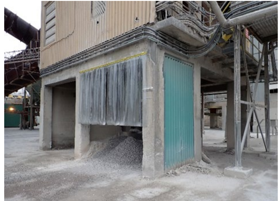
December 2018: Kiln #2 Smoke Chamber Fallout area enclosed
