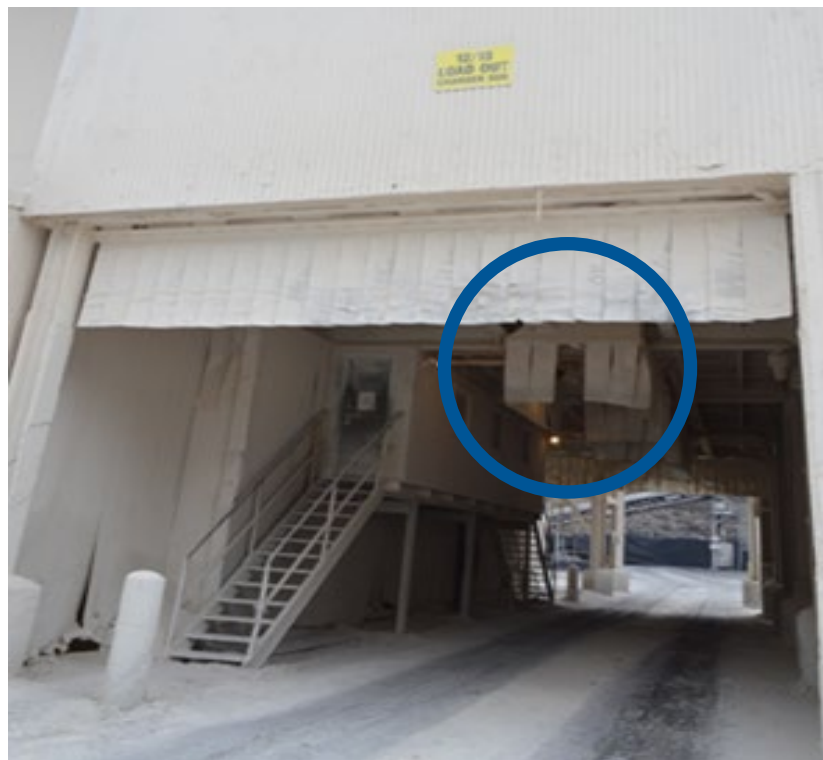
December 2015: Bin 12/13 Loadout with damaged dust curtain (plastic strips)
