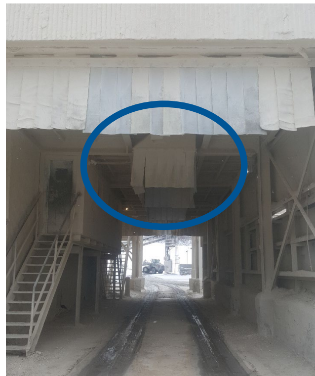
February 2021: Bin 12/13 Loadout area dust curtains
