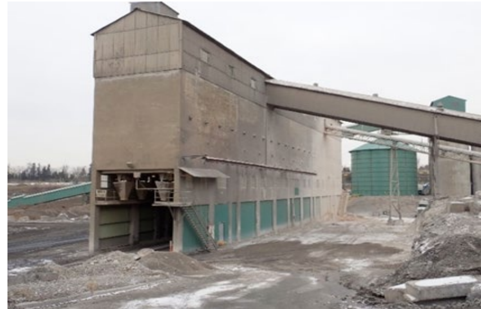
December 2018: Bunker Loadout area enclosed with metal sheeting and pile of lime removed
