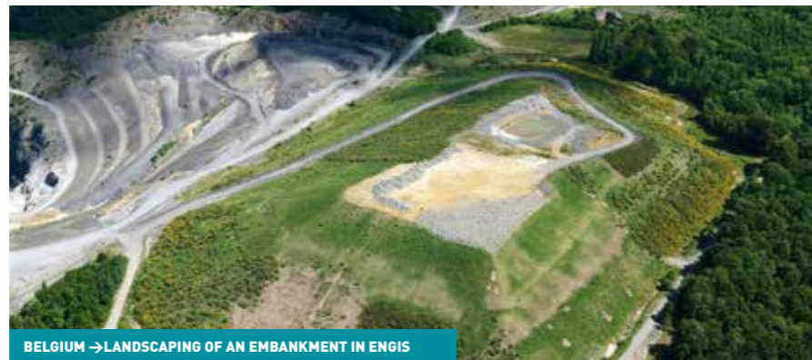
BELGIUM → LANDSCAPING OF AN EMBANKMENT IN ENGIS
